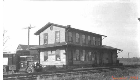
Former Southampton Railroad Station. c. 1920
