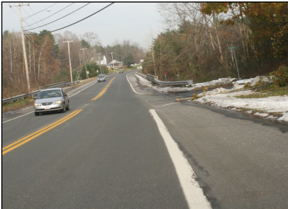
Route 10: Wide shoulder versus narrow limited shoulder
